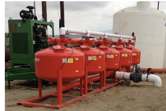
Containerized slow sand filters
