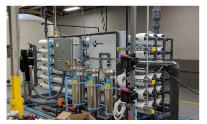
**Pre-Treatment/Pre-filtration**: Removing organic and organic debris, including plant material, sediment, and algae.
